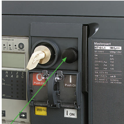
Electrical closing pushbutton BPFE.
